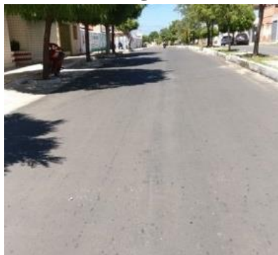
(a) Trecho 4 – Centro 1
